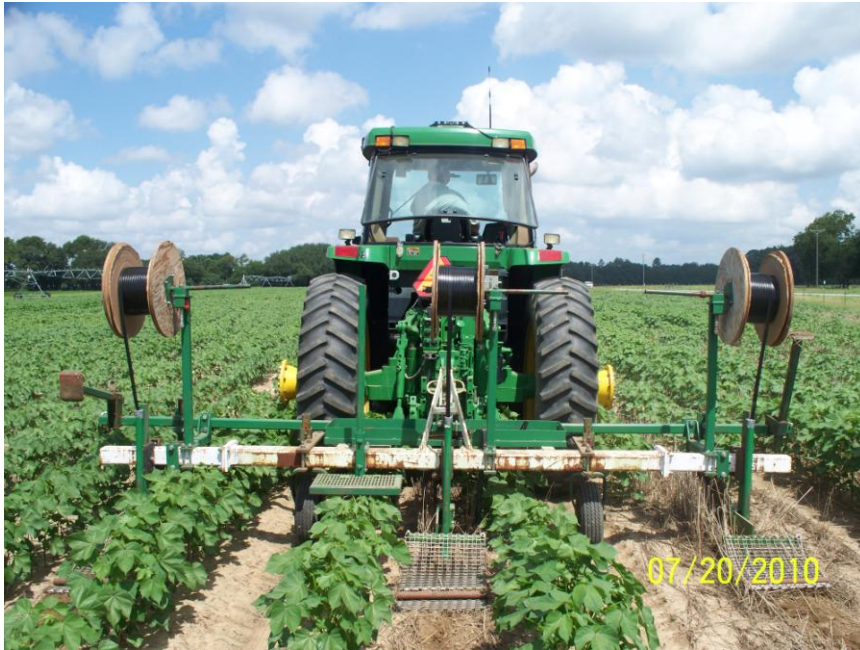
Installing SSDI drip tape – July 20, 2010.
