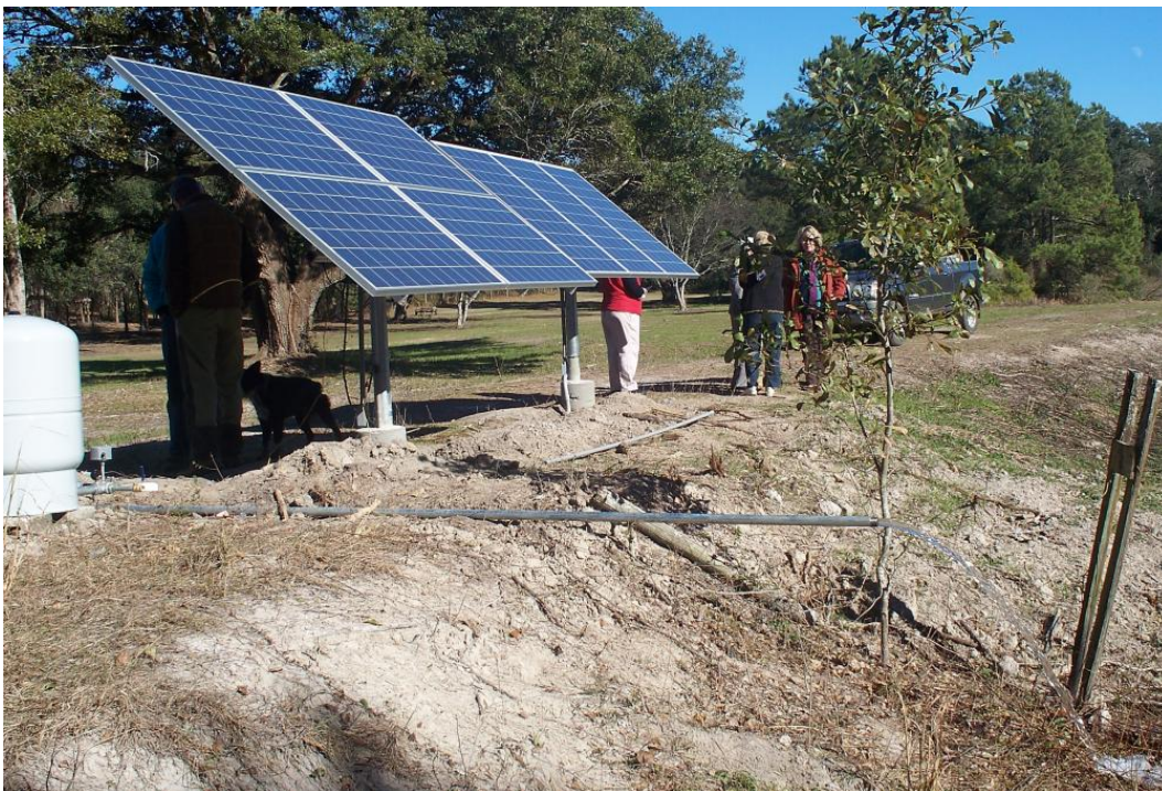
The Stripling family's new solar-powered well supplying water to one of their ponds.
